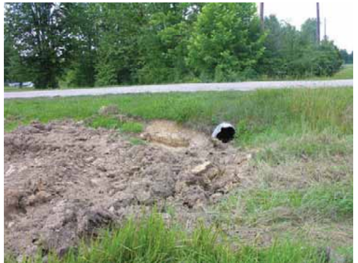
Photographs 5-6. The lot located at wagon Wheel Dr. and Indian Dr. had no silt fence installed. This culvert (right) drains runoff from the lot to Cove 4.
