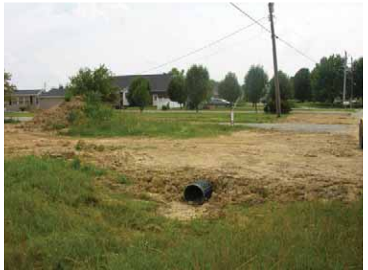
Photographs 29-30. The drainage area to Cove 11 has many developing lots that lack sediment and erosion control.
