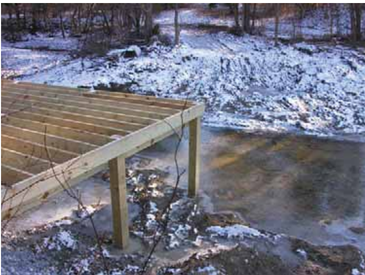
Photographs 11-12. This dock, located at the head of Cove 6, was installed over winter 2011. No erosion or sediment controls were used during installation.
