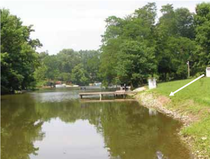
Photographs 3-4. The shoreline is eroding (indicated by white arrows in photos) at the upstream end of Cove 4 (Kiddie Corral).
