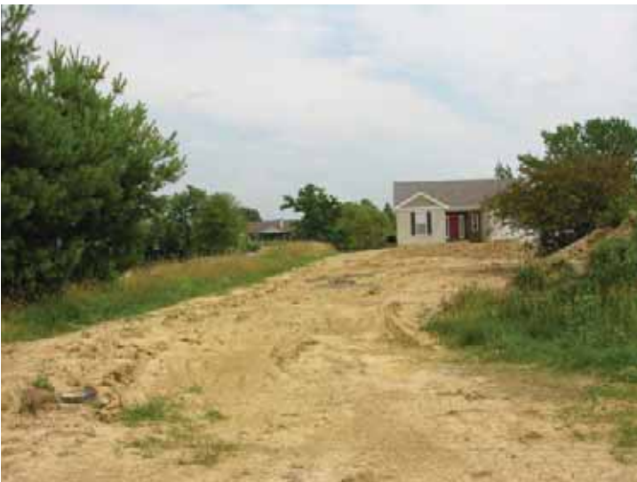
Photographs 29-30. The drainage area to Cove 11 has many developing lots that lack sediment and erosion control.
